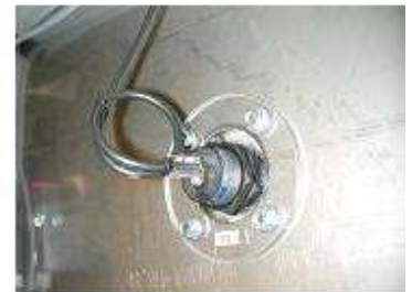
Liquid tank level" sensor
