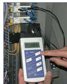
The programming of the ASiBus addresses is done with a specific addressing terminal (Option)
