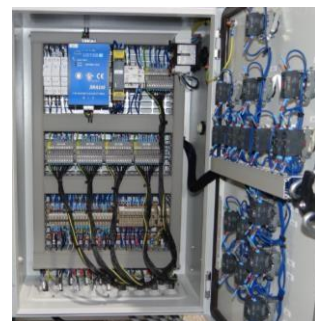
Electrical box with standard and plug-in terminal blocks
